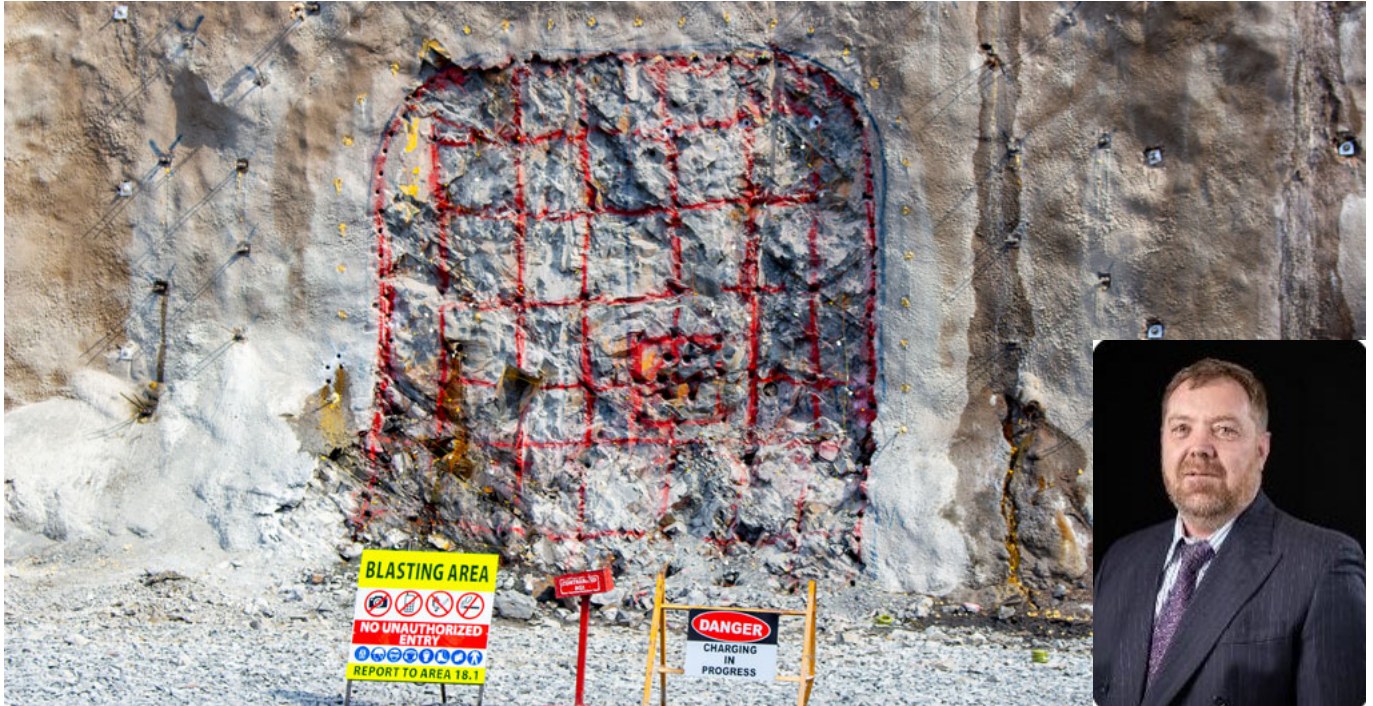
↑ One of the three portals earmarked for blasting
